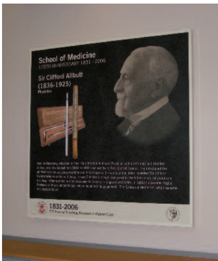
Wall hung OWAcoustic Broadband absorbers on the lower level provide an efficient acoustic absorber hidden behind a work of art and, on the upper level, as a colour co-ordinated absorber providing a more subtle aesthetic effect.
