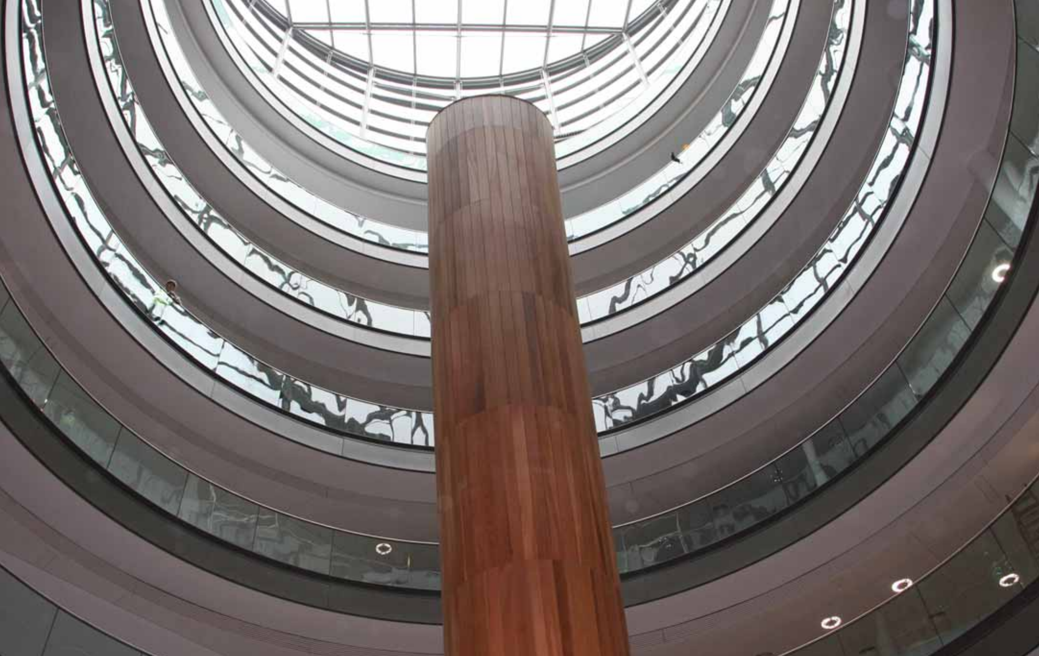
Spandrel Panels, Riverside One, Dublin
