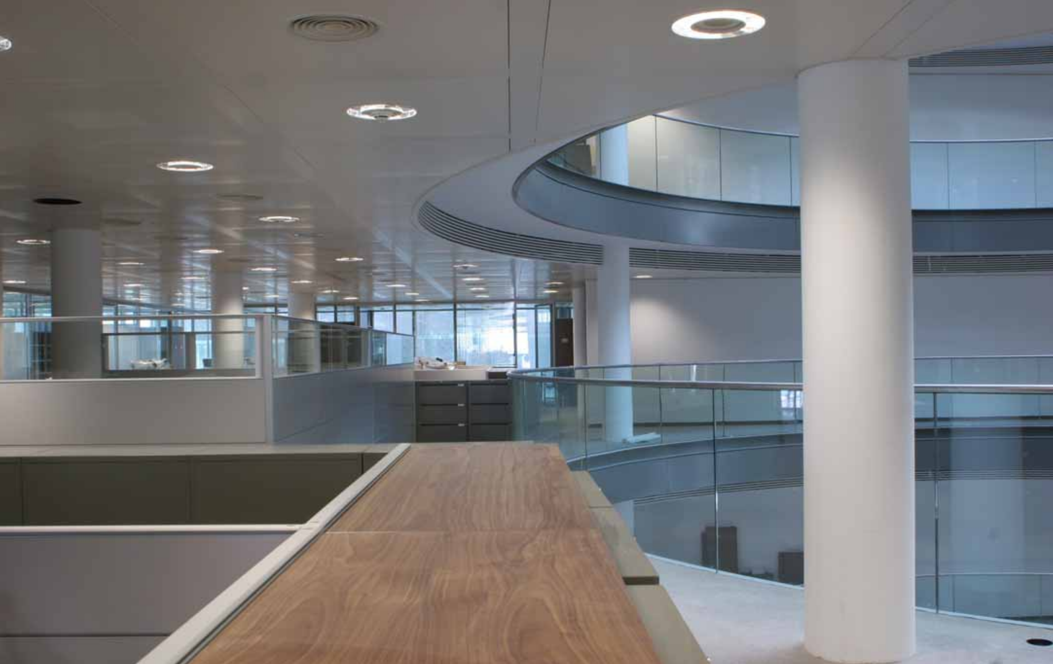
Spandrel Panels, Riverside One, Dublin
