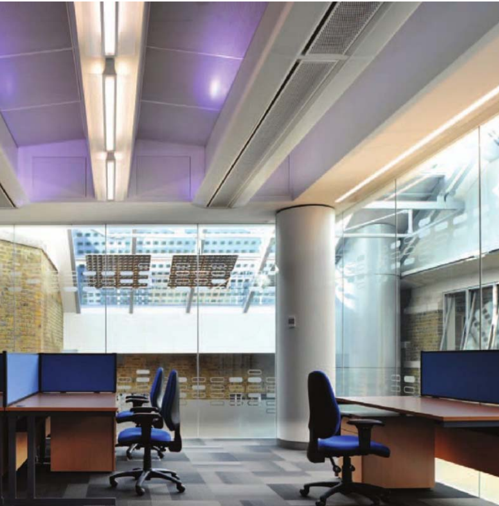
By combining an internal summer temperature with chilled beams, larger reductions in a building's running costs can be achieved.
